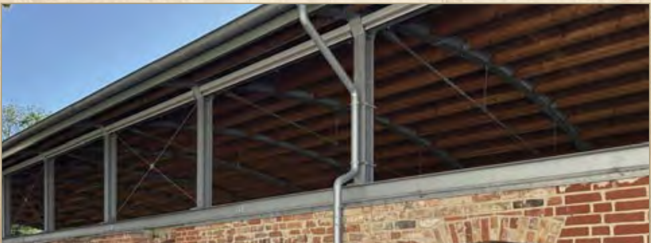
Weather protection blinds at the Altfriedland Monastery Ruin
