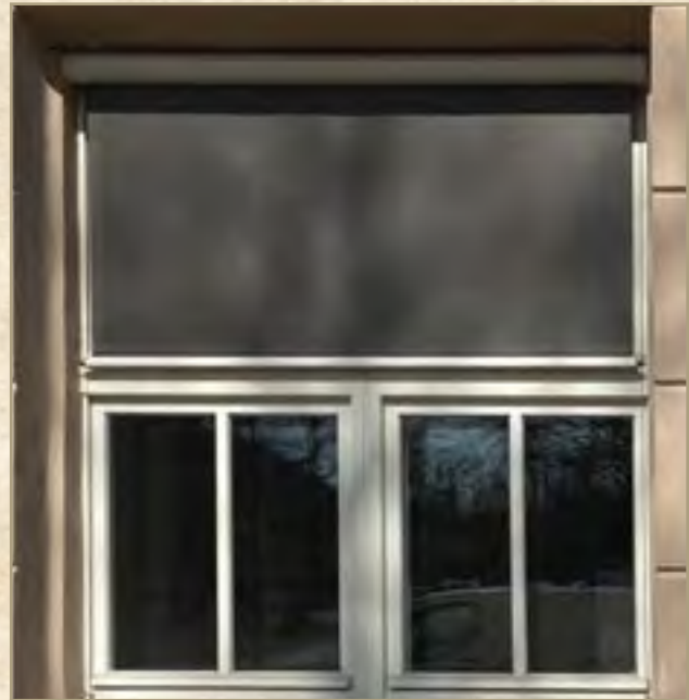
Exterior view (7.3 cm casing, mounted in the reveal)
